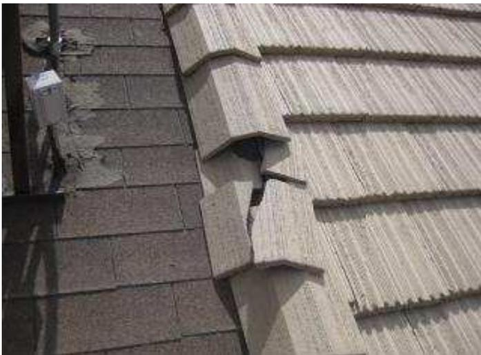
View of cracked tile at west facing roof slope next to asphalt shingle roof to AC/Heat pump.
