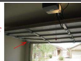
**N.W. side of home Garage Service Doors:** Fire rated, self closing Self closing door does not fully self close and latch. Recommend licensed contractor adjust self closing hinges so that it fully closes and latches for fire safety precautions.
